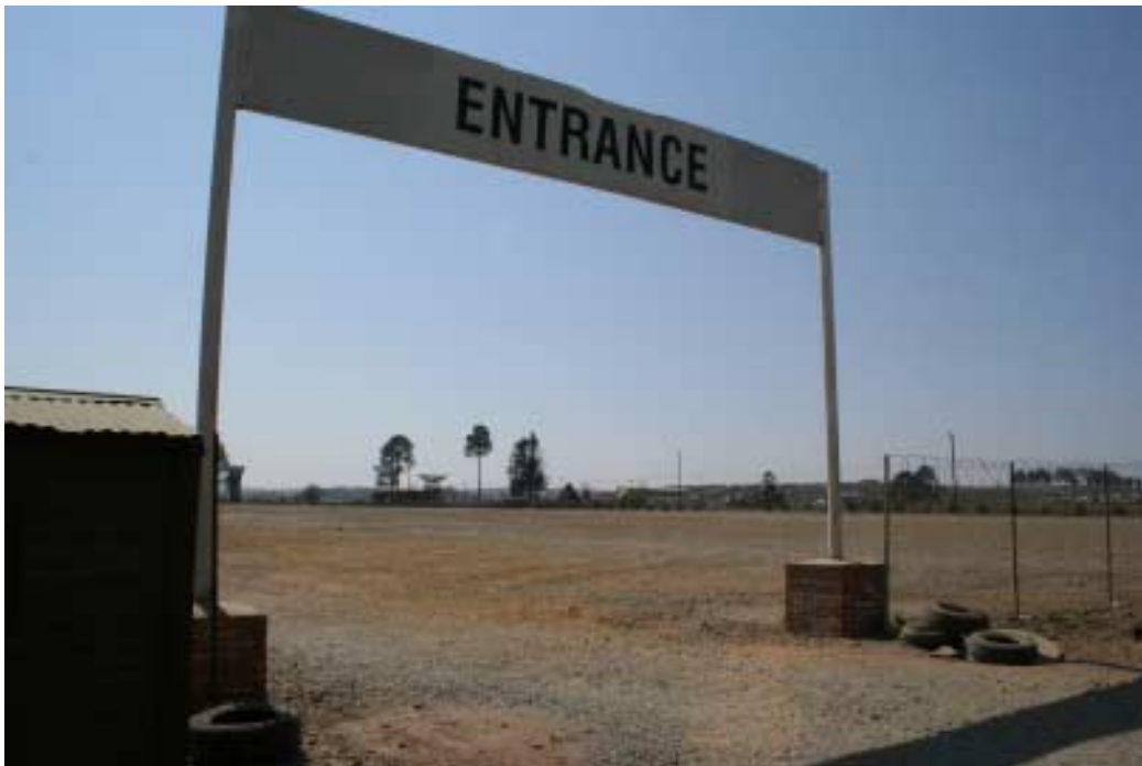
Figure 2 Entrance lane at Mooi River Truck Stop
