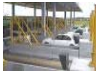
Toll station (S.Africa)
